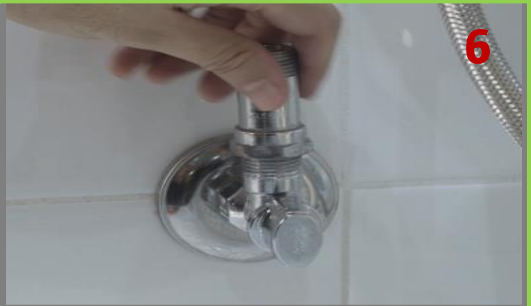
Connect Dual Check Valve to Water Tap
