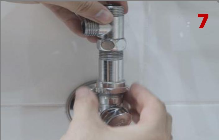
Connect T-Piece Adaptor to Dual Check Valve
