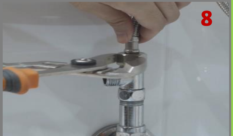
Connect Braided Hose to T-Piece Adaptor
