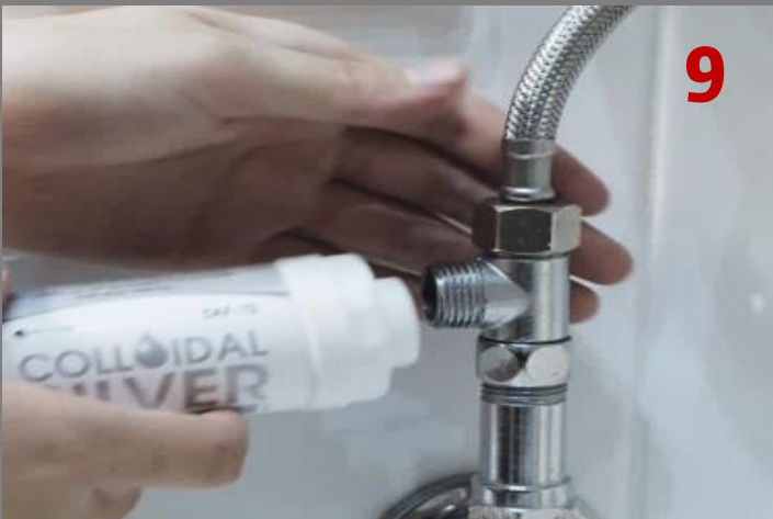
Connect Filter to T-Piece Adaptor
