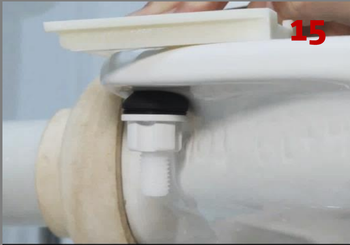
Insert Seat Bolts Through Sliders Into Bolt Holes
