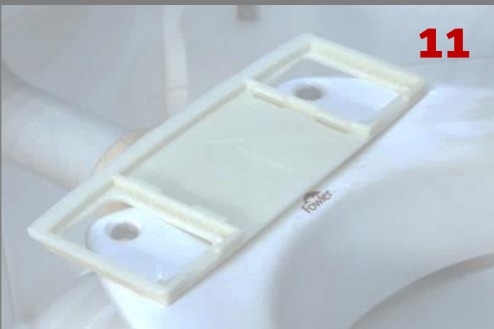
Place Base Plate on Toilet Pan
