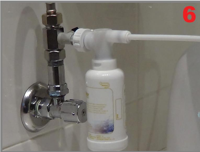
Insert filter and twist clockwise.
