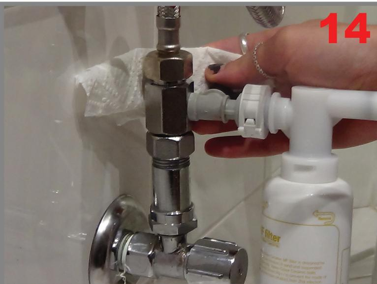
Turn on water check for leaks with a piece of toilet paper. Tightened joints if required.
