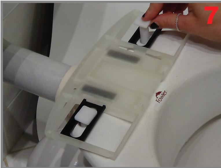
Place installation plate on toilet, place bolts through
