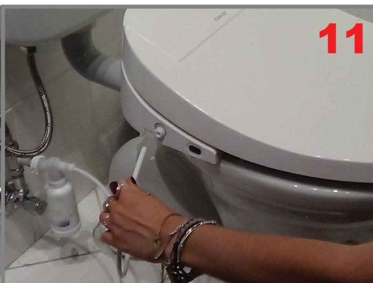
Push Bidet pipe into hole on left hand side of Bidet.
