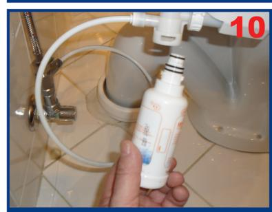
Insert MF filter into filter holder and turn to the right to secure.
