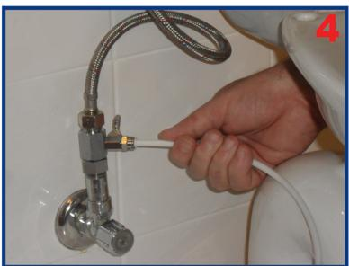
Push white pipe into T-Piece. This is a John Guest fitting and needs to be inserted securely.
