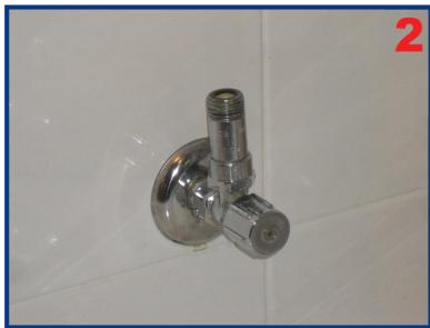
Install Backflow valve (Dualcheck) with green washer on water supply.
