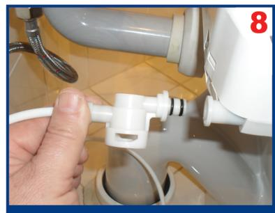
Insert white pipe into filter holder then push holder into the back of the bidet.
