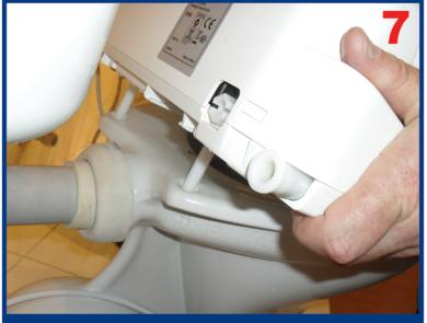
Place bidet onto toilet and set in position, now install and tighten nuts with supplied tube spanner.
